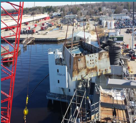
Old Stack being removed
